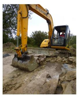
To begin with as each section of liner was cut out the digger dragged it up the slope and piled it up on the other side of the fence.
